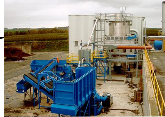
Preparation and drying
